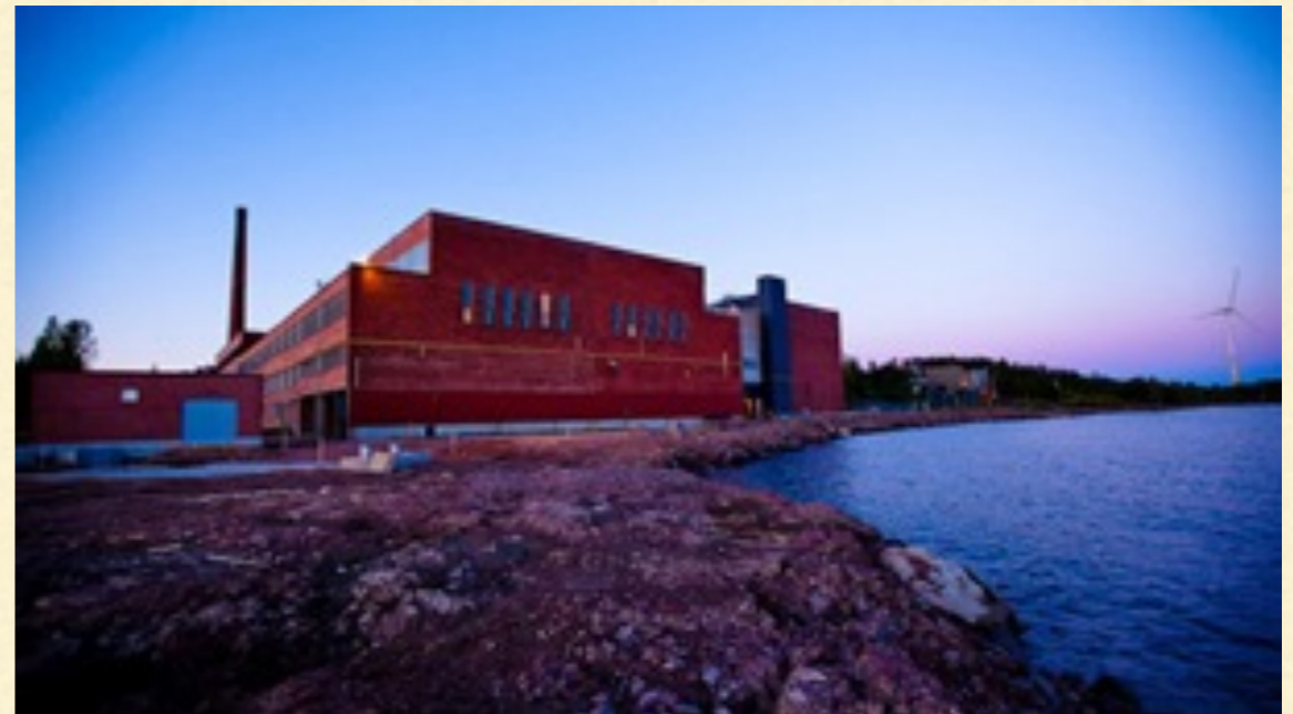
Google data center in Hamina, Finland
