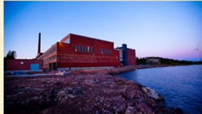
Google data center in Hamina, Finland
