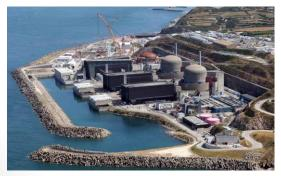
Most powerful nuclear reactor under construction in France: Flamanville (EDF, 2017 for 10 billion €) 1650 MW
